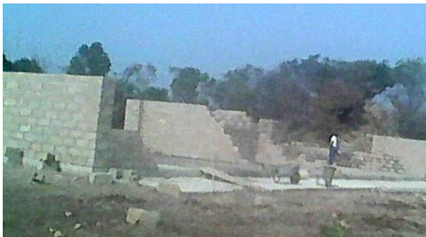
3-classroom block under construction
