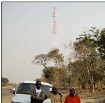
New cellular telephone tower near Lumwana West
