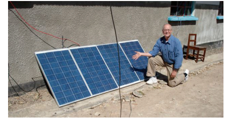
Gerry displays the solar panels
