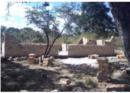
Librarian's house under construction.
